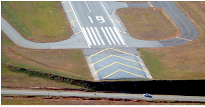
Photograph of an EMAS installation (The EMAS bed is the grey area under the yellow chevrons)
